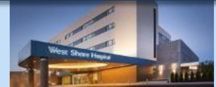
West Shore Hospital
